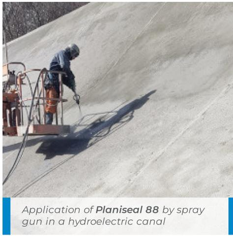
Application of Planiseal 88 by spray gun in a hydroelectric canal
