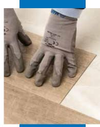
Installation of LVT with Ultrabond Eco V4 Evolution
