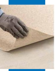
Installation of homogeneous PVC with Ultrabond Eco V4 Evolution
